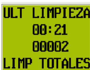
Last backwashing & total backwashings screen image
